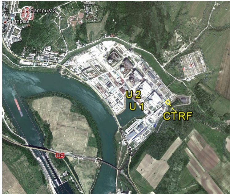
Fig. III.1 CTRF location within Cernavoda NPP site
