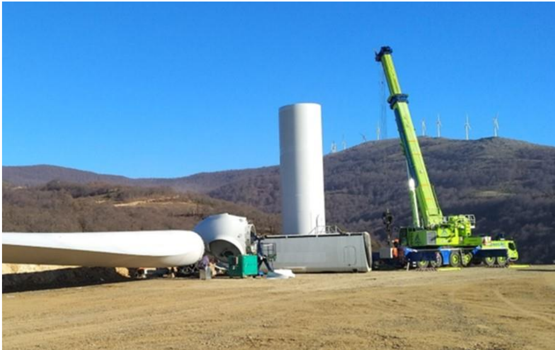
Image from 1: Erection of the W/T (indicative photo)
