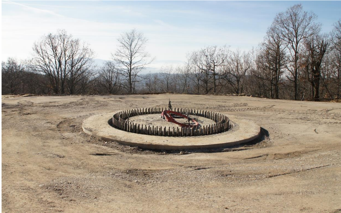
Image from 9: Foundation of the W/T
