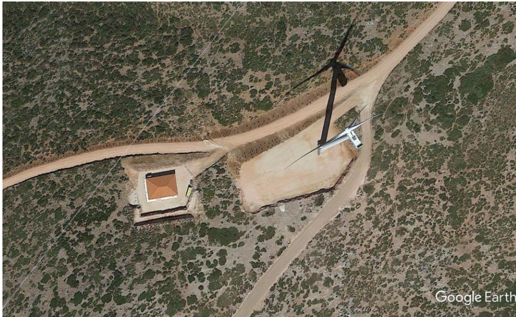
Image from 10: Panoramic View of a Typical Control Tower in a Wind Farm
