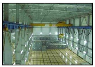
FIGURE 2.2-5 TEMPORARY STORAGE IN THE STORAGE FACILITY FOR STORAGE OF CONDITIONED RAW ON THE SITE OF NPP KOZLODUY
